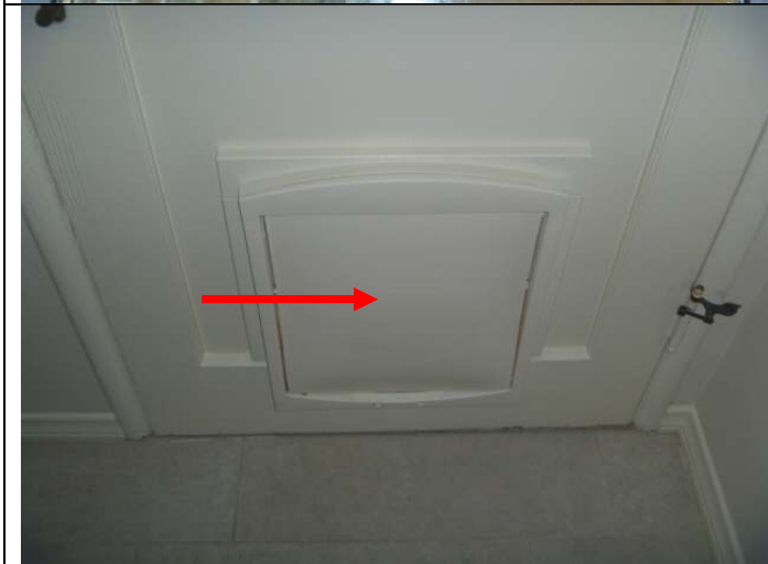
Pet door in the service porch exterior door.
