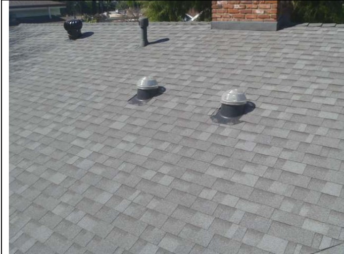
Composition shingle roofing.
