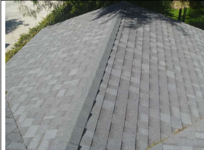
Composition shingle roofing.
