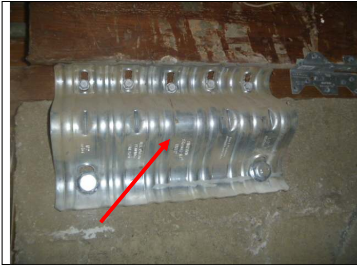
Retrofit foundation anchor plate.
