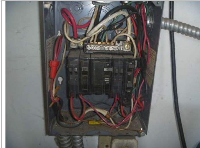
Lower subpanel on the garage rear wall.
