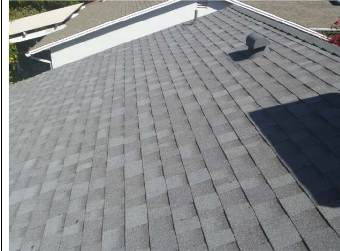
Composition shingle roofing.
