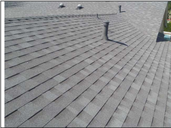
Composition shingle roofing.
