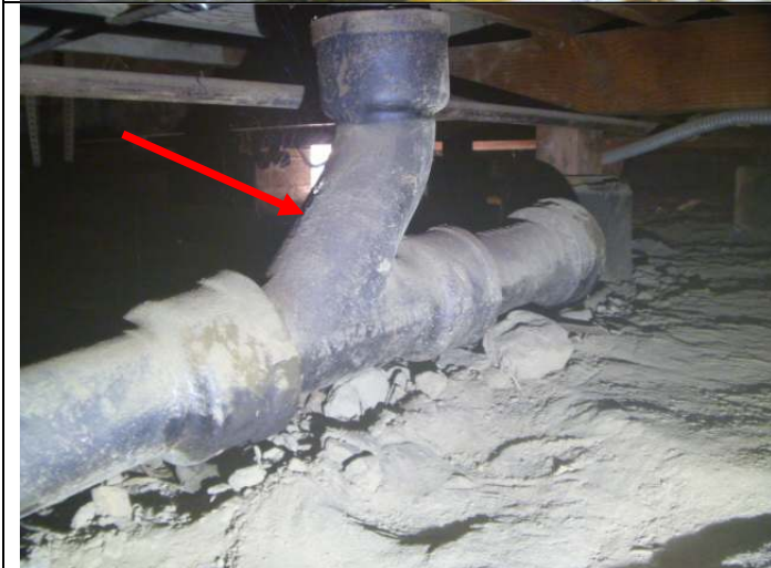
Original cast iron drain piping.
