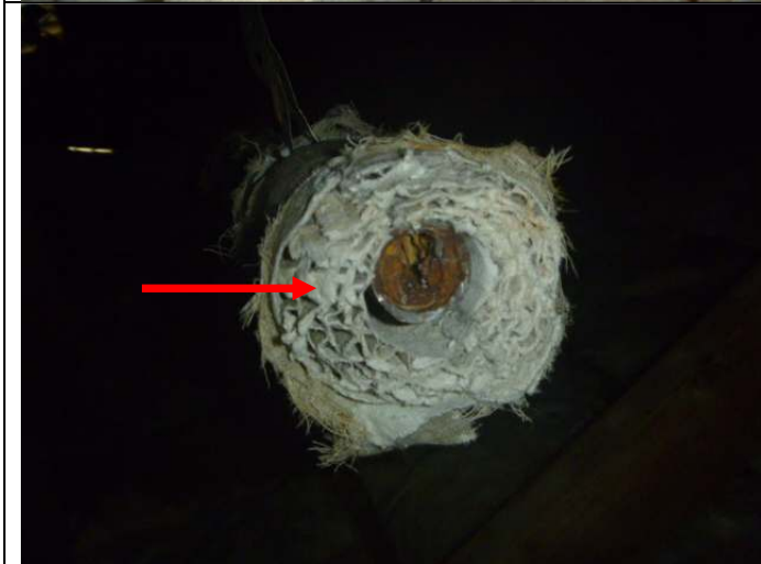
Cross section of the above noted asbestos pipe insulation.
