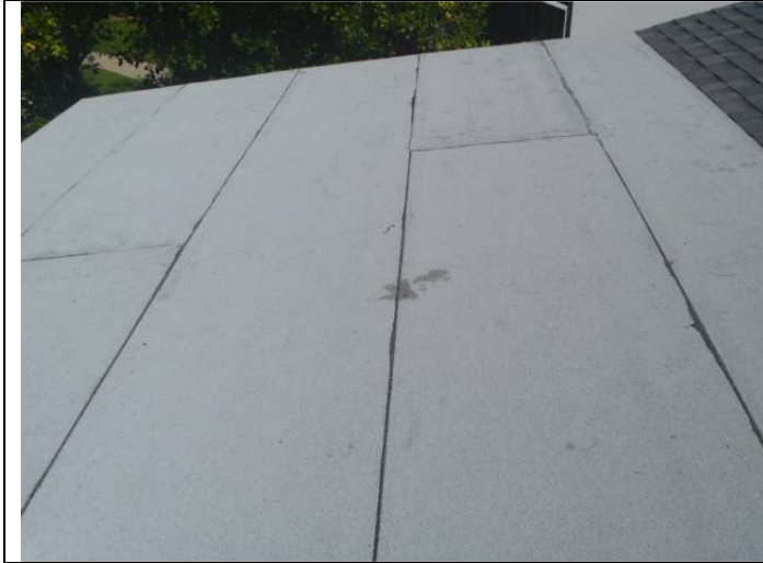
Rear patio covering roof.
