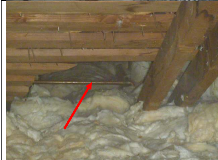
Limited access to the far right front attic area.
