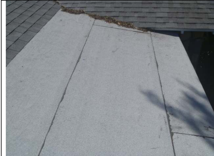
Rear patio covering roof.
