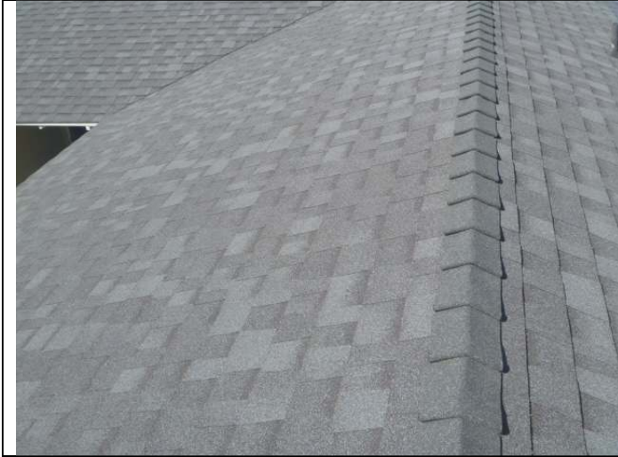
Composition shingle roofing.
