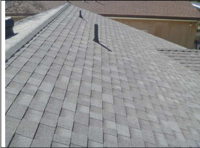
Composition shingle roofing.
