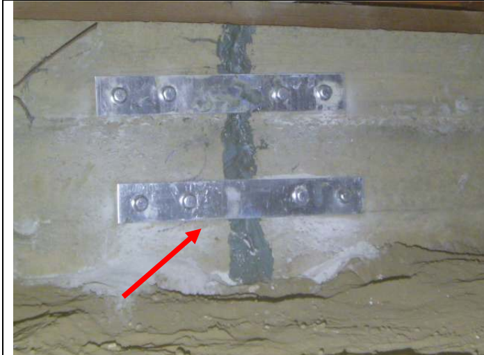
Foundation crack repair (toward the right front).
