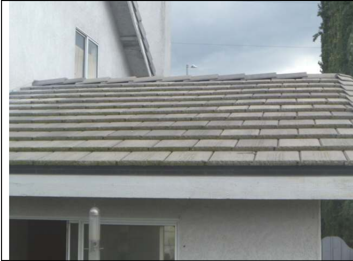
Tile roofing (lower left rear).
