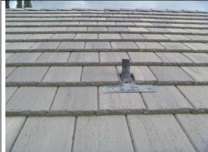
Tile roofing (upper rear).
