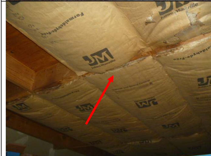
Fiberglass insulation on the unfinished sunroom ceiling.
