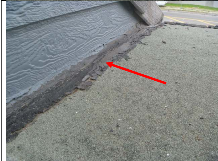
Sealant along the perimeter of the above roof.
