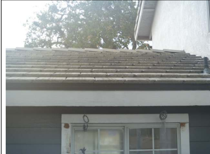
Tile roofing (lower left front).
