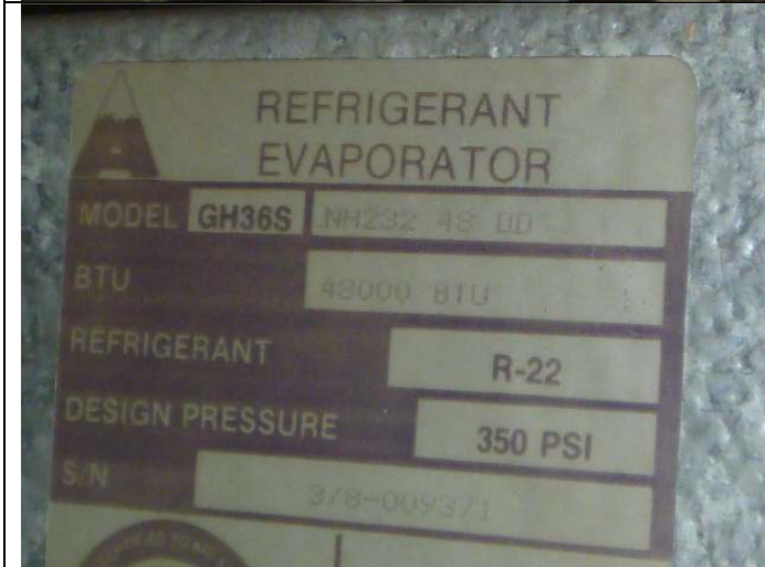
Air conditioner coil model number, capacity, refrigerant type (R-22) and serial number.
