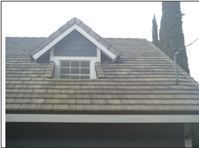
Tile roofing (upper front).
