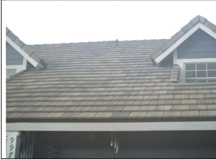
Tile roofing (upper front)
