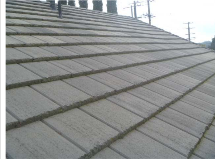
Tile roofing (upper rear).
