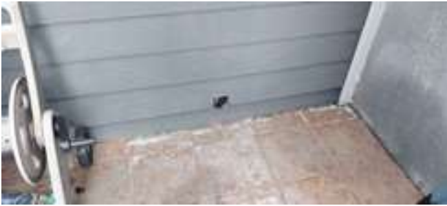
Additional small wall cleanout. Not used for today’s inspection.
