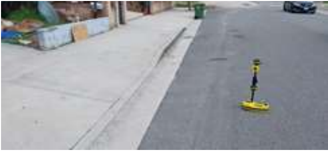
Connection to city sewer line. Depth about 6’.
