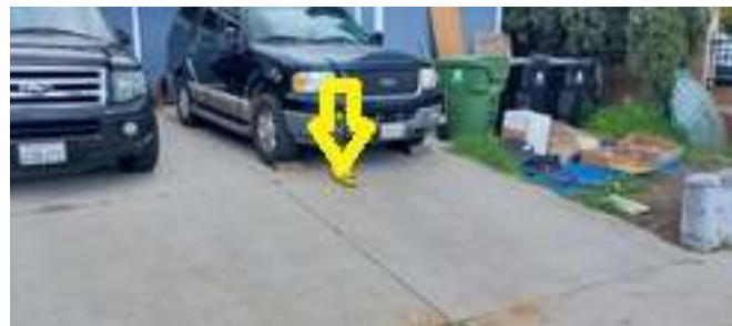
Transition from plastic to clay pipe. Depth about 5 1/2'.
