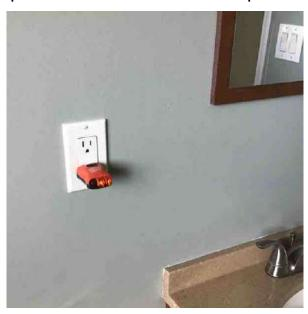
8.7.4 The receptacle(s) are miswired (reversed polarity, open neutral, etc.) A qualified electrician should correct as required for electrical safety. (Bedroom Two)
