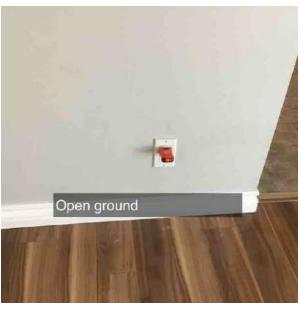
8.7.2 Open Neutral. The receptacle(s) are miswired (reversed polarity, open neutral, etc.) A qualified electrician should correct as required for electrical safety. (Master Bedroom)
