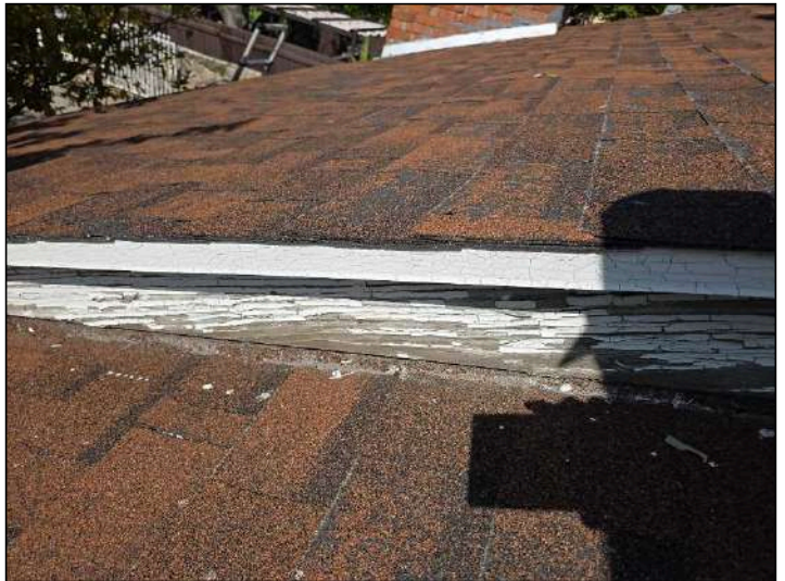
Missing sidewall flashing, recommend repair
