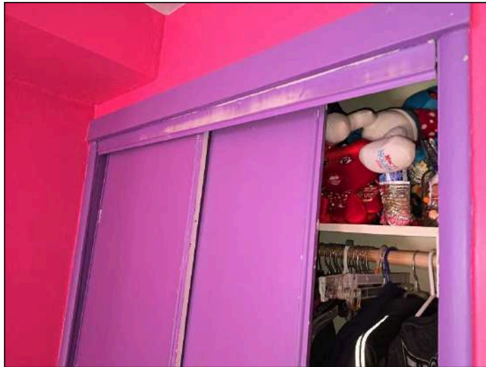
Doors off tracks and heavily worn east bed
