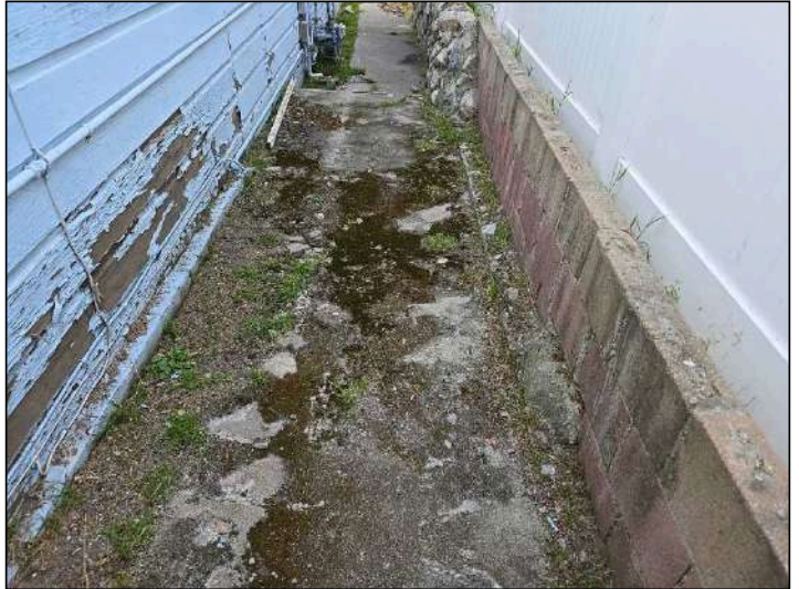
Stains present, evidence of ponding water east side, recommend further evaluation
