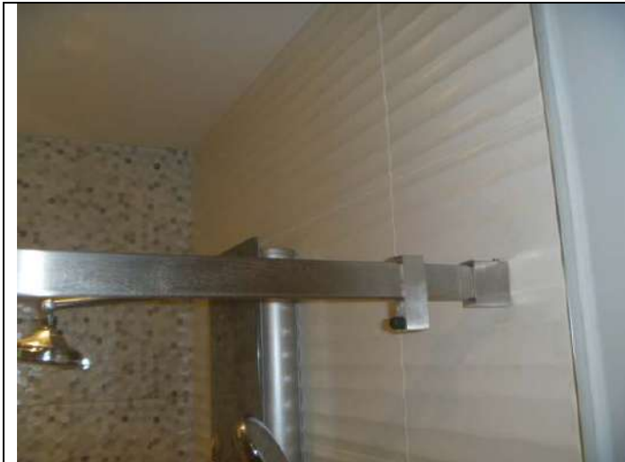
ADU shower. Note: The tiles backing type was not determined.
