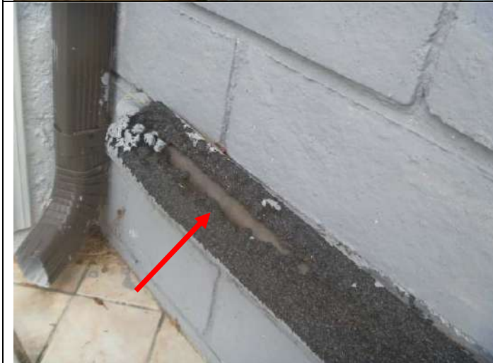
Surface mounted water piping to the ADU.
