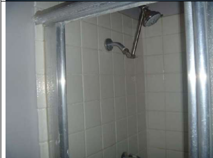
3/4 bathroom shower. Note: The tiles backing type was not determined.
