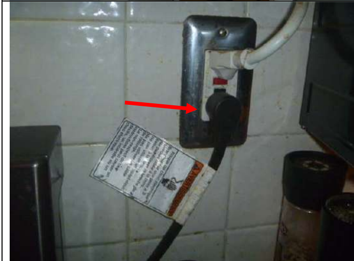
Range/oven plugged into the countertop area receptacle to the right of the range/oven.
