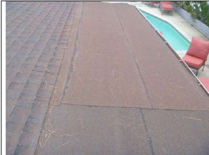
Rear patio covering roof.
