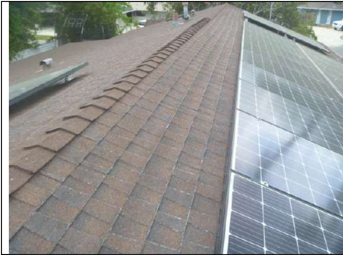
Composition shingle roofing.
