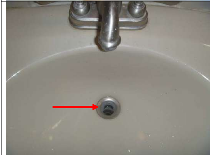
Full bathroom sink with missing stopper.
