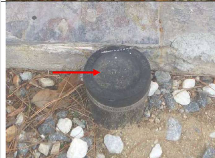
Drain cleanout at the right front of the front porch.
