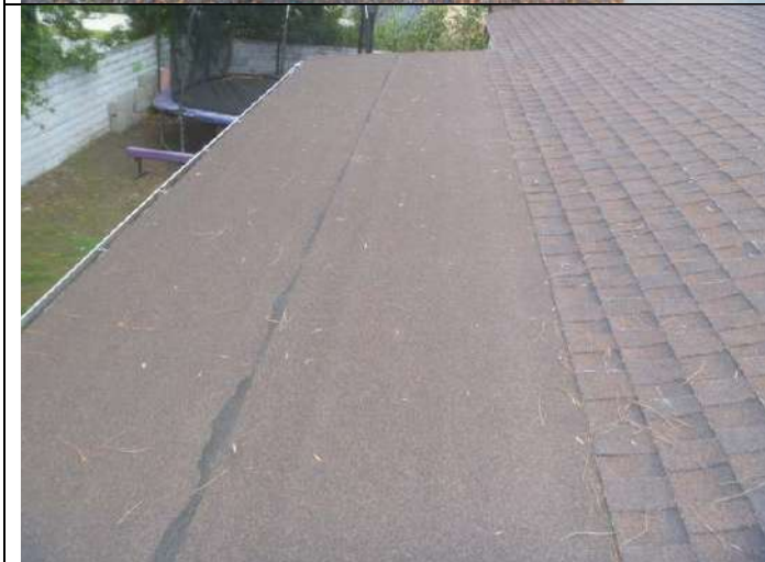
Rear patio covering roof.
