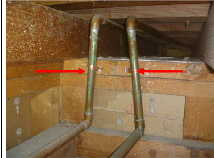
Replacement copper water piping routed through the attic.
