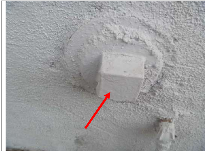
Drain cleanout at the lower right front exterior wall.
