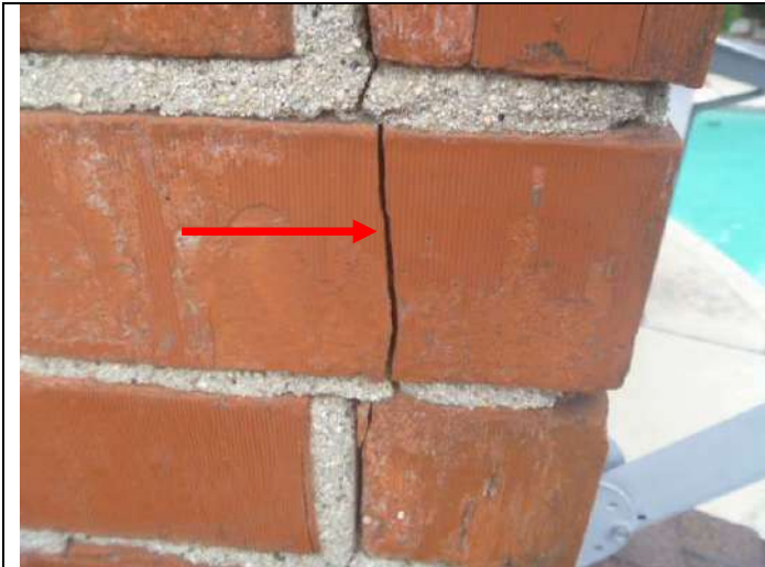
Chimney cracking.
