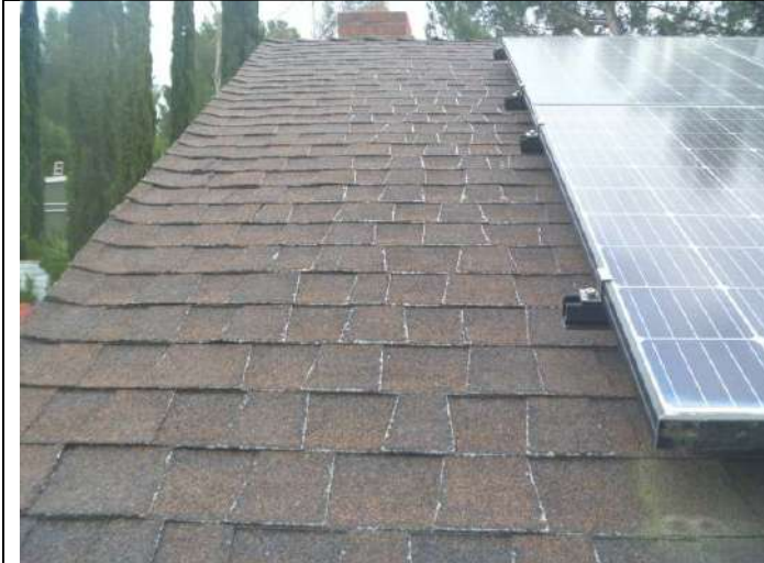
Composition shingle roofing.
