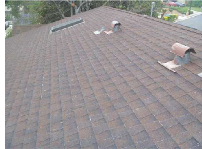
Composition shingle roofing.
