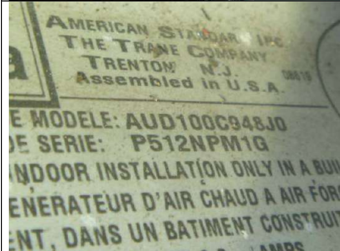
Heater/fan unit model and serial numbers (possibly indicating a 1999 build date).
