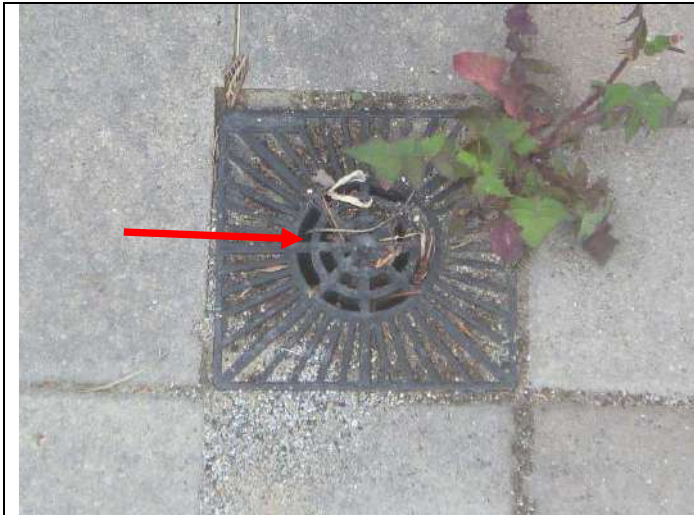
An exterior surface drain.
