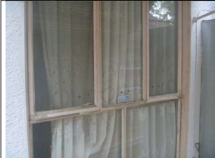
Example of older windows (off the rear bedroom).
