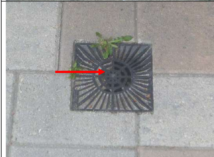
An exterior surface drain.
