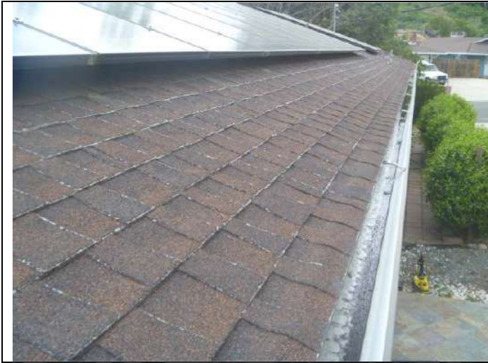
Composition shingle roofing.
