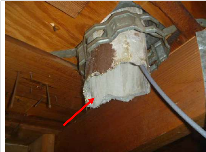
The above noted vent pipe visible in the attic.
