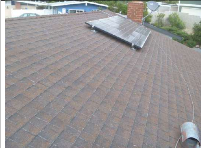
Composition shingle roofing.
