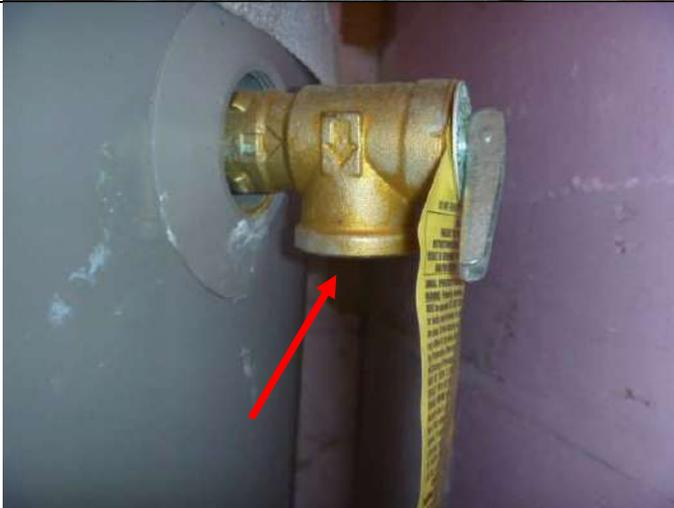
No drain pipe for the pressure relief valve on the water heater.
