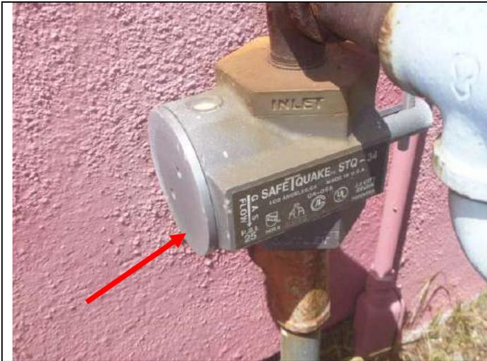
Older seismic shut off valve for the gas piping.
