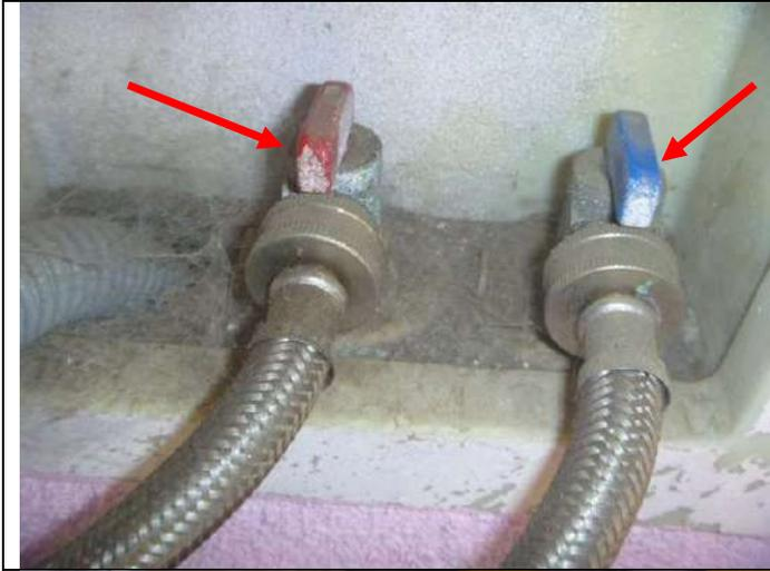
Washer valves. Note: The valves are stuck or stiff (not forced).
