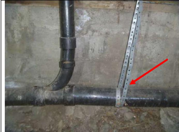
Replacement ABS drain piping braced with metal (vs. nonmetallic) strap.
