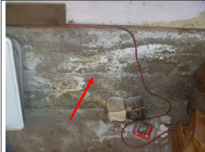
Evidence of moisture along the garage lower interior wall.
