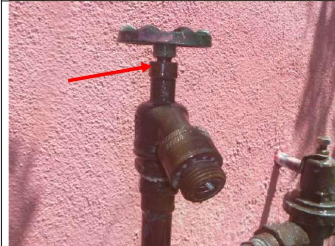
Front exterior hose bibb (which leaks during operation).
