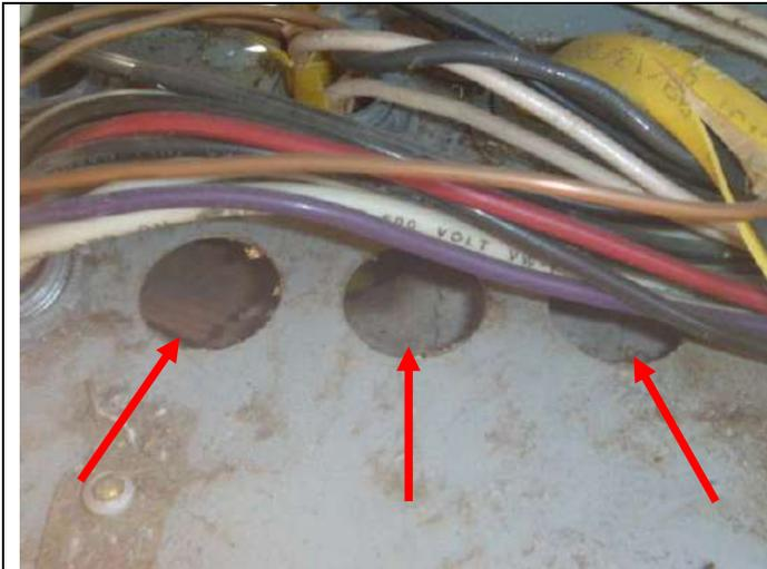
Open knockouts in the base of the panel cabinet.
