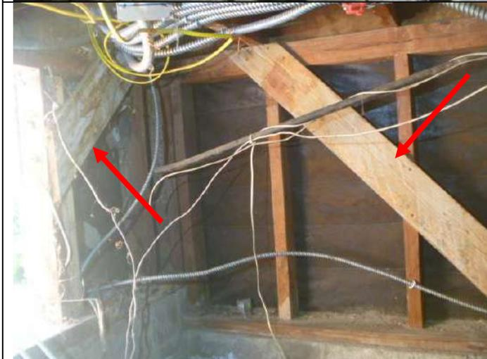
Foundation cripple stud wall with original diagonal type bracing.
