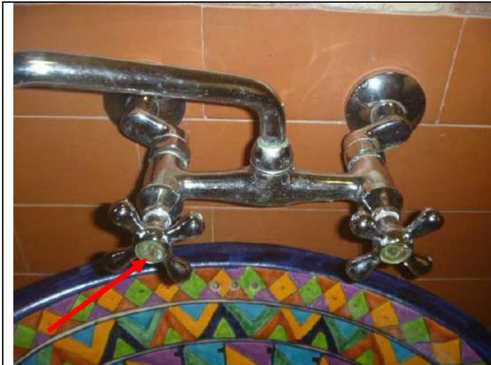
Full bathroom sink faucet. Note: The hot water valve turns past the roof position.
