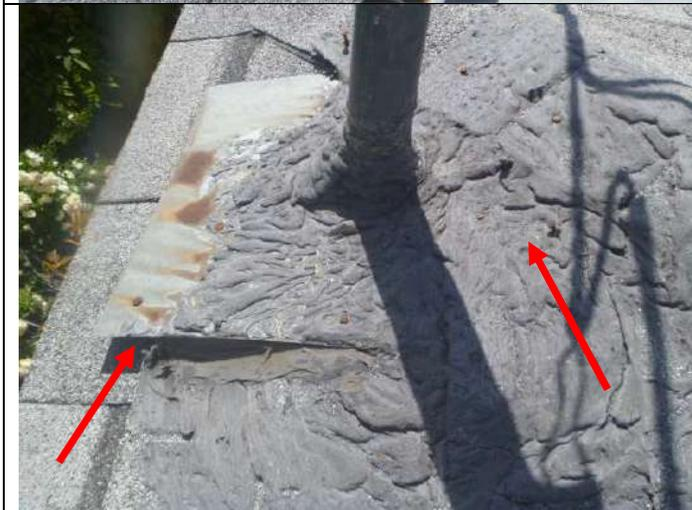
Lifted flashing and irregular sealant at the electrical service entrance.
