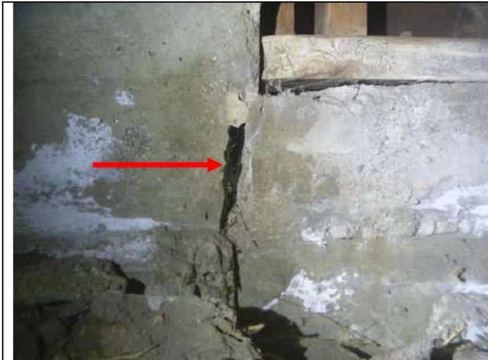
Crack in the foundation south wall.
