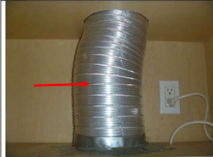
Flexible (vs. rigid) duct above range hood.
