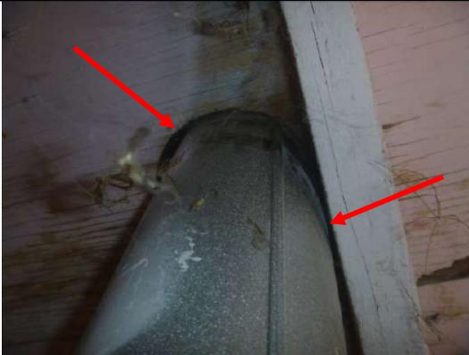
Water heater vent pipe without the proper wood clearances at the rafter and roof sheathing.
