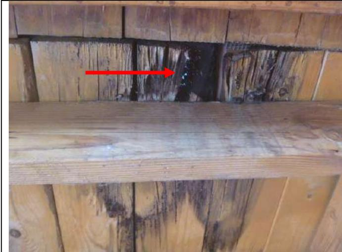
Damaged wood on the underside of the rear patio covering roof.
