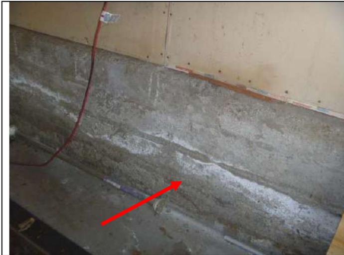
Evidence of moisture along the lower interior wall.
