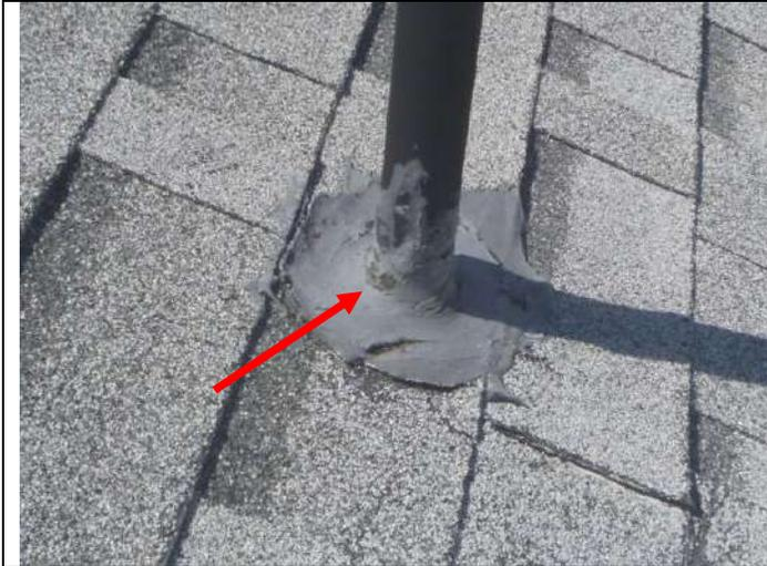
Plumbing vent pipe without a visible flashing at the left rear (over the kitchen).
