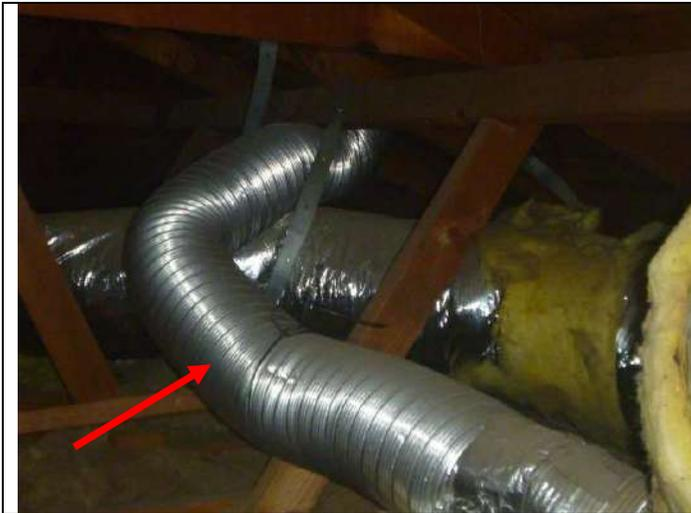
Range hood flexible (vs. rigid) and long vent duct in the attic.
