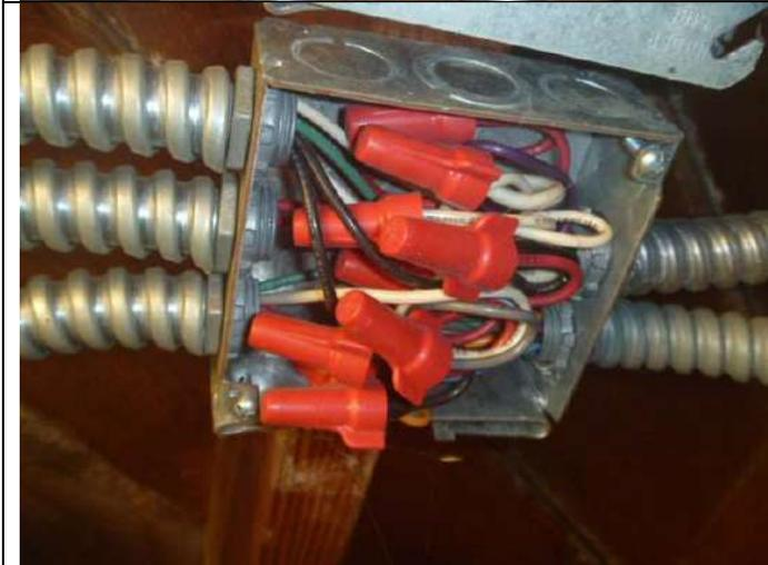
Open electrical box in the foundation crawlspace.
