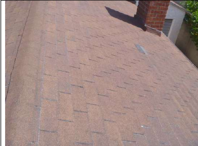
Composition shingle roofing.
