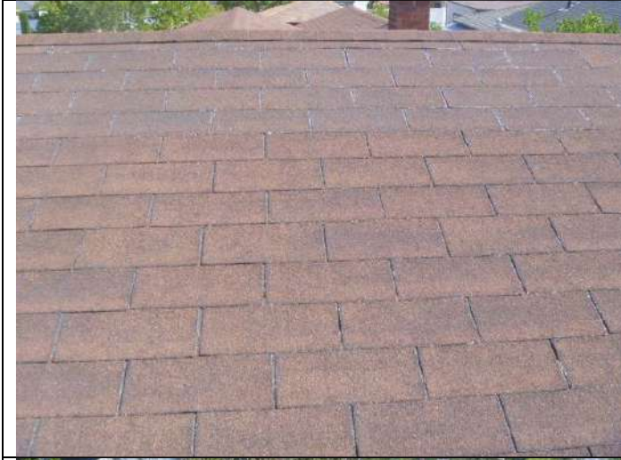
Composition shingle roofing.
