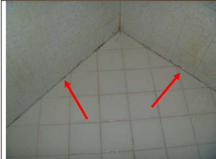
3/4 bathroom shower pan. Note: There is sealant along the base of the walls.
