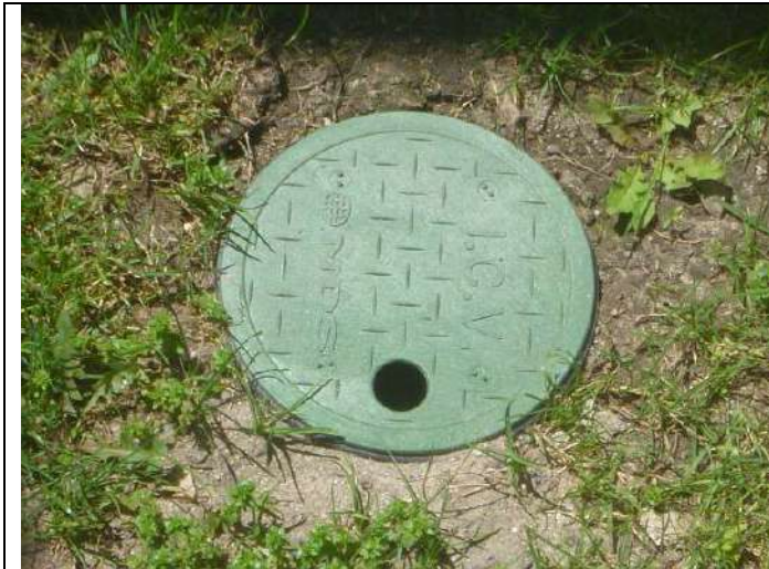
Drain cleanout at the left rear exterior.
