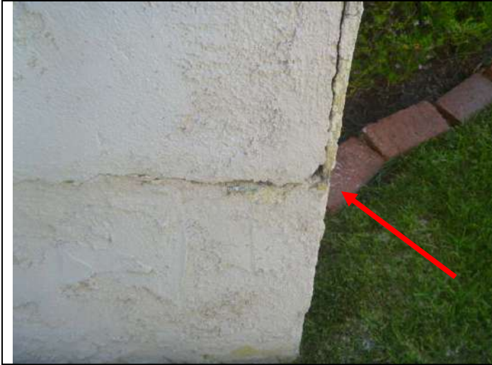
Stucco cracking.
