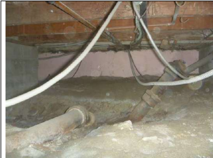
Left rear addition foundation crawlspace.
