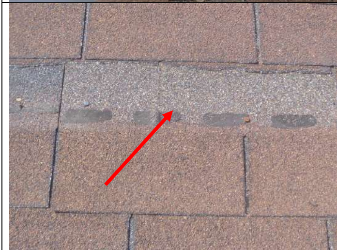
Missing shingles.
