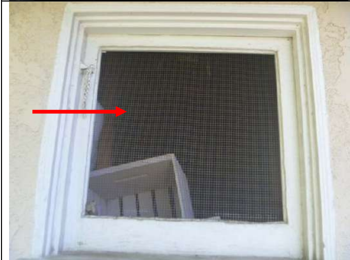
Garage window with screen (vs. a window pane).
