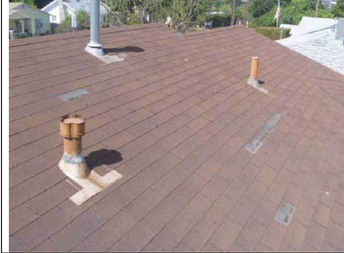
Composition shingle roofing.
