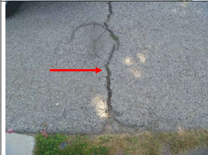
Driveway cracking.
