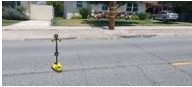
Connection to city sewer line. Depth about 14'.
