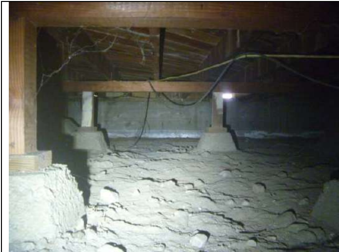
Main foundation crawlspace.
