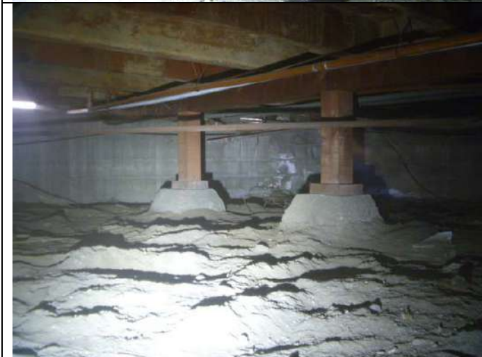
Main foundation crawlspace.
