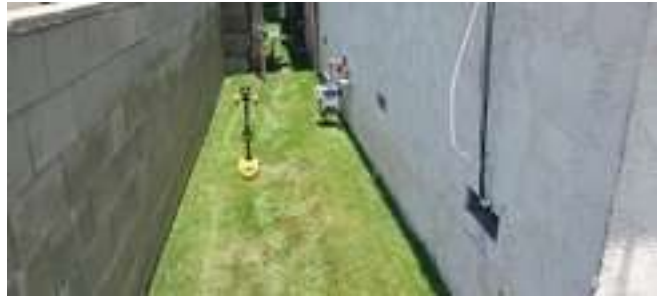
Path of pipe along side of house. Depth about 4'.
