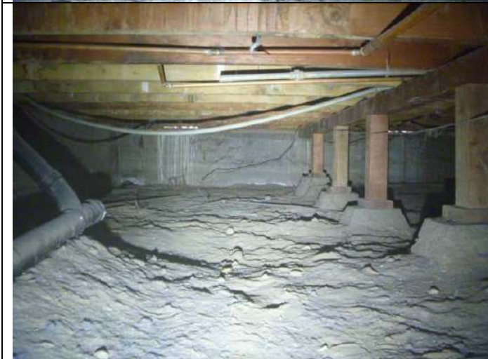
Main foundation crawlspace.
