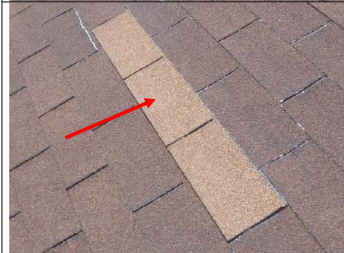
Replaced shingles.
