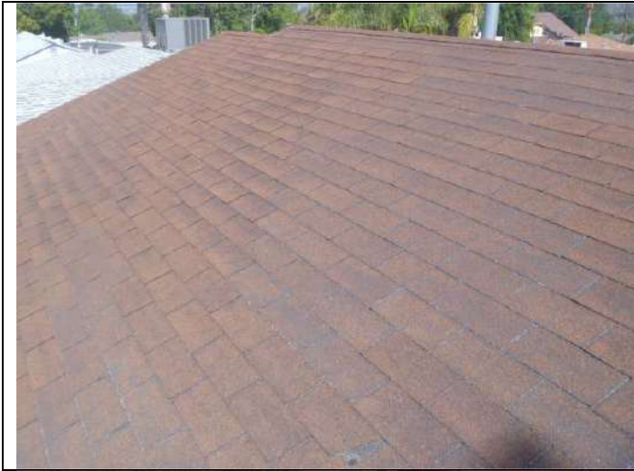
Composition shingle roofing.
