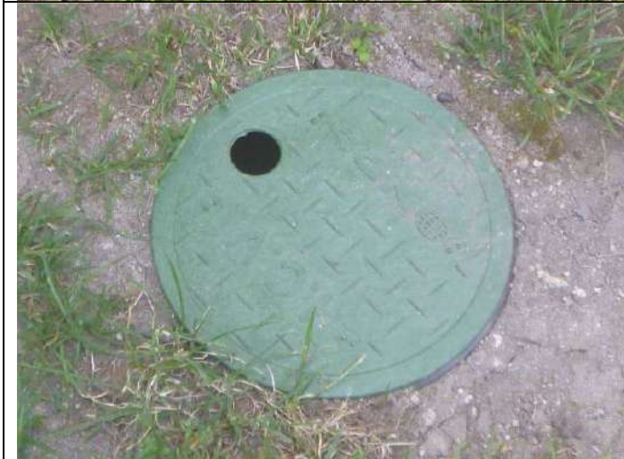
Drain cleanout at the left rear exterior.
