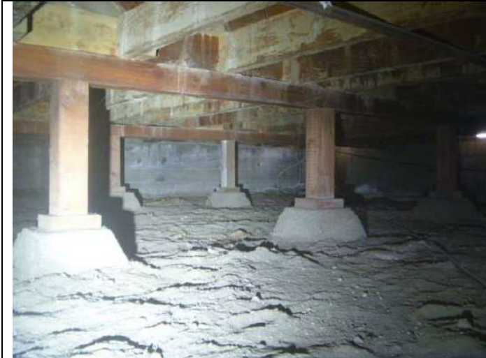
Main foundation crawlspace.
