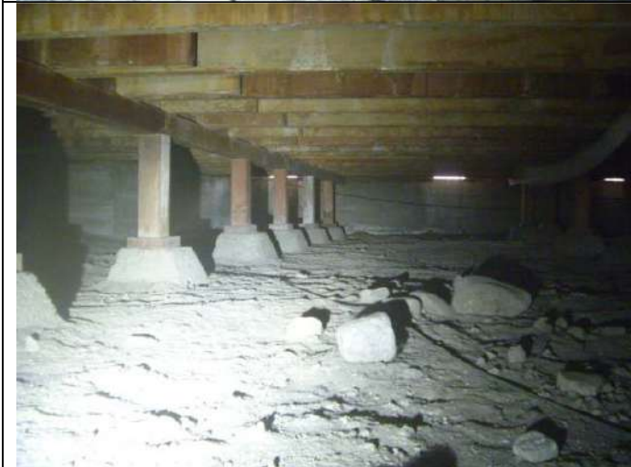
Main foundation crawlspace.
