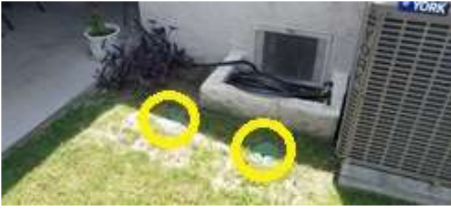
Cleanout behind house.
