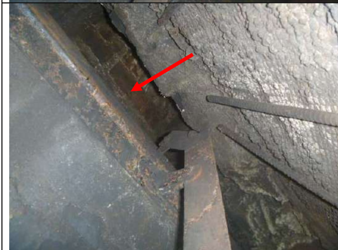
Fireplace damper in the open position.
