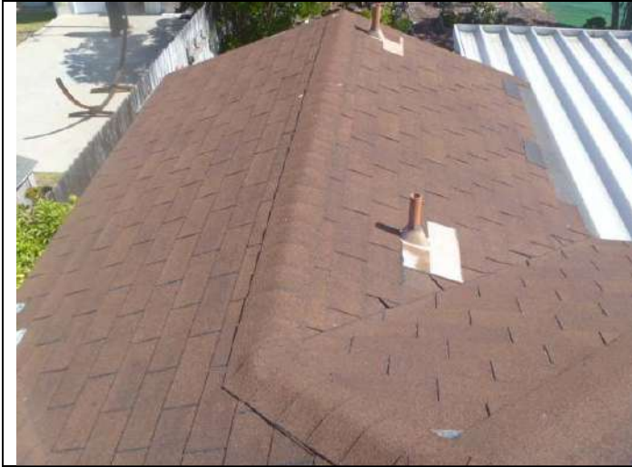
Composition shingle roofing.
