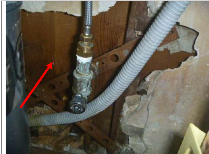
Opening in the wall below the kitchen sink.
