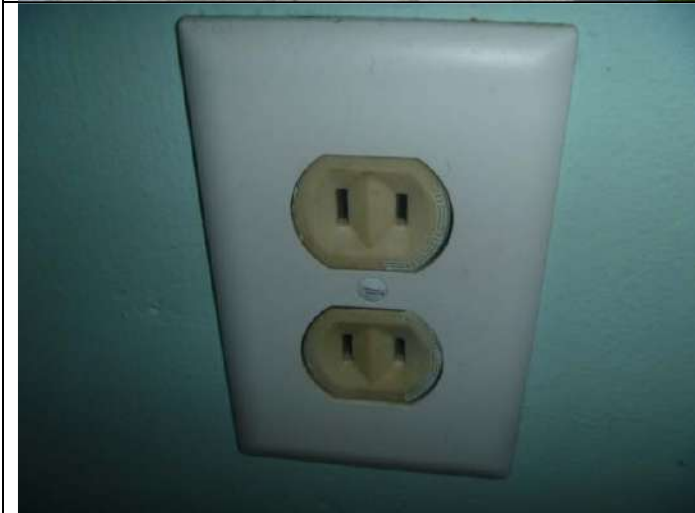
Example of an older receptacle.
