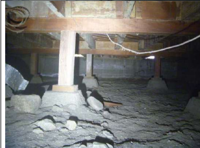
Main foundation crawlspace.
