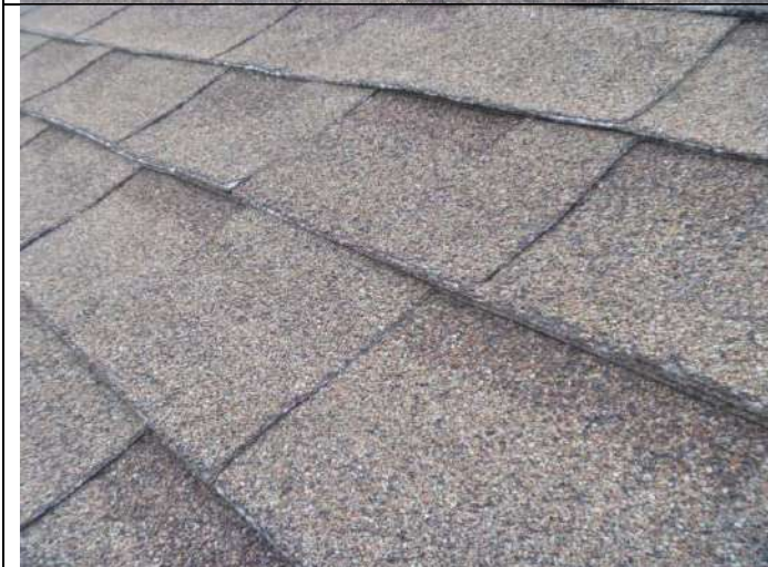
Older shingle close-up.
