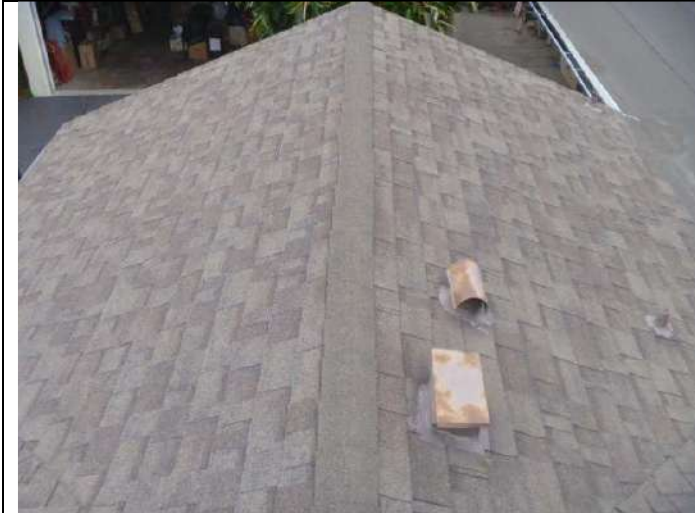
Composition shingle roofing.
