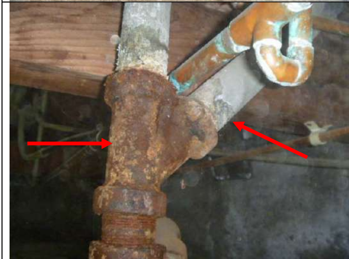
More original drain piping.
