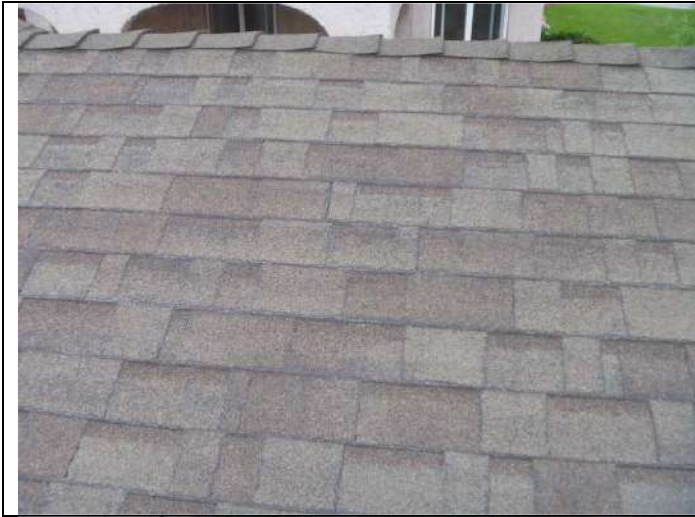
Composition shingle roofing.
