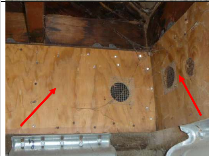
Retrofit plywood bracing for the perimeter cripple stud walls.
