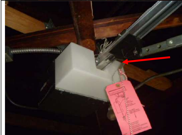
Garage door opener (screw drive type).
