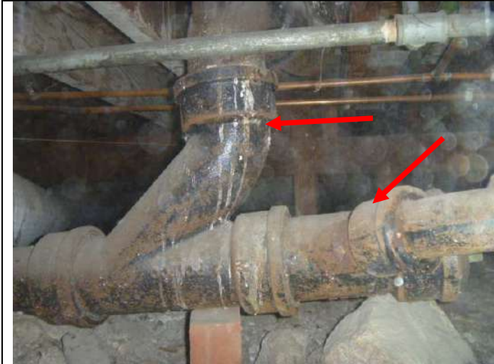
Example of original drain piping.
