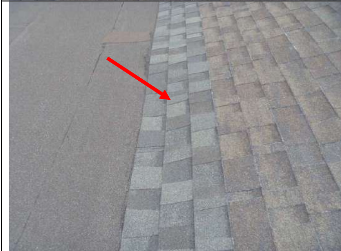
Newer shingles along the flat roof transition.
