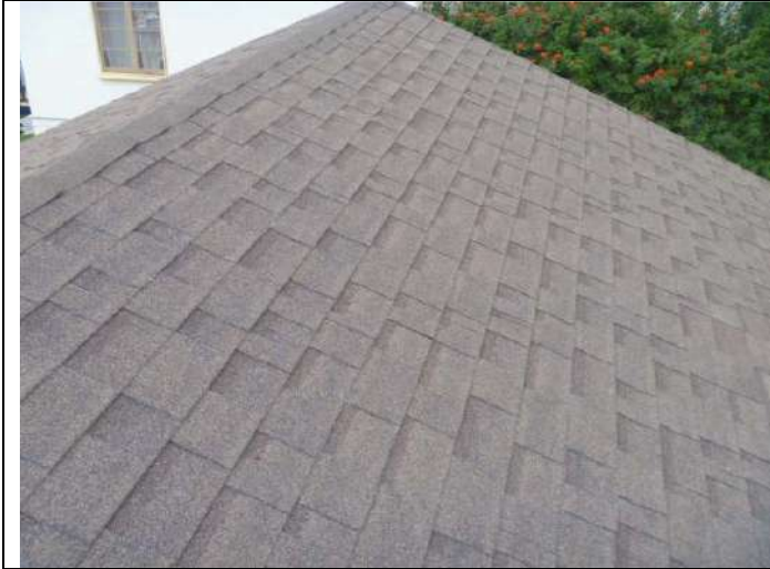
Composition shingle roofing.
