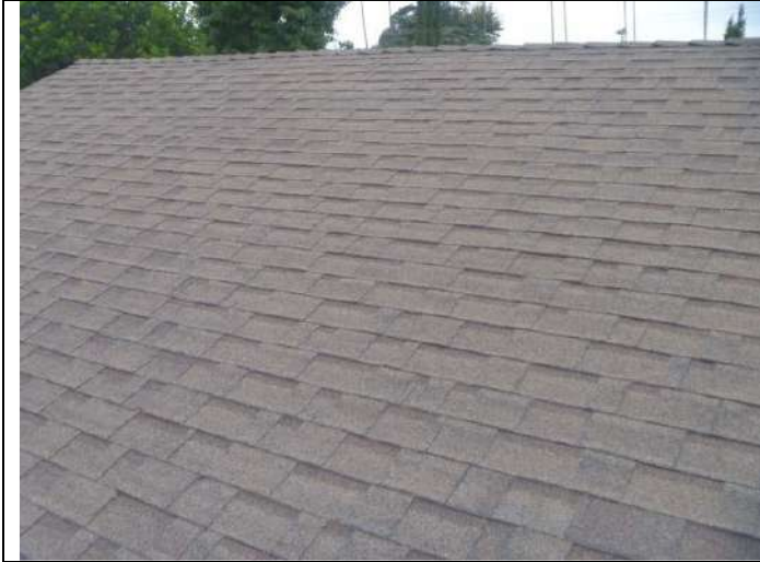
Composition shingle roofing.
