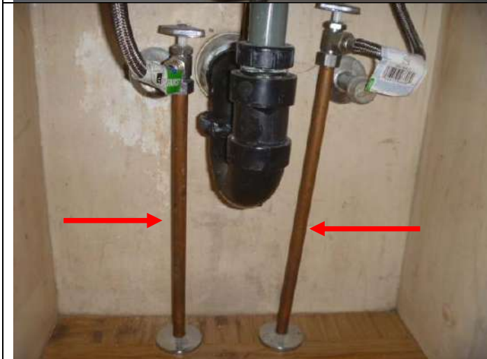
Surface mounted replacement water piping below the front bathroom sink.
