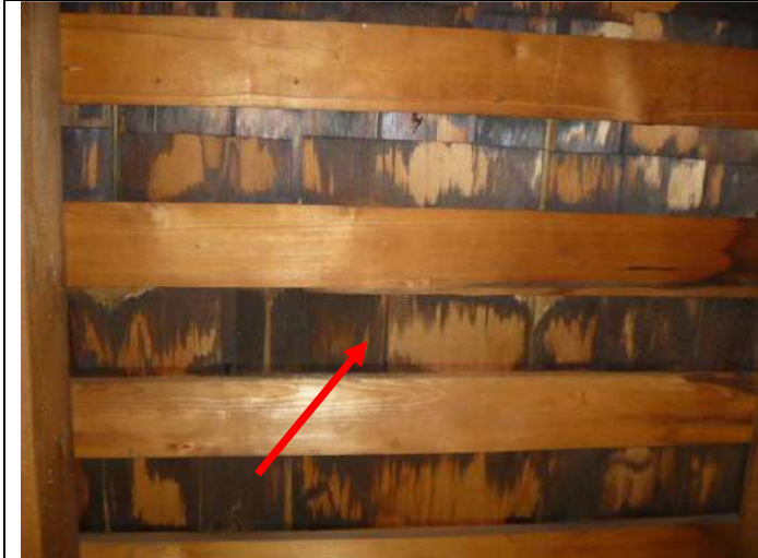
Original wood shingle roofing under the composition shingles.
