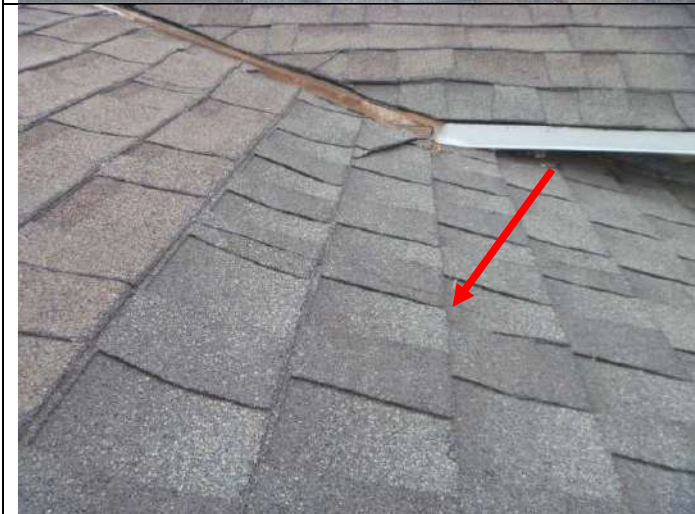
Newer shingles over the front porch.
