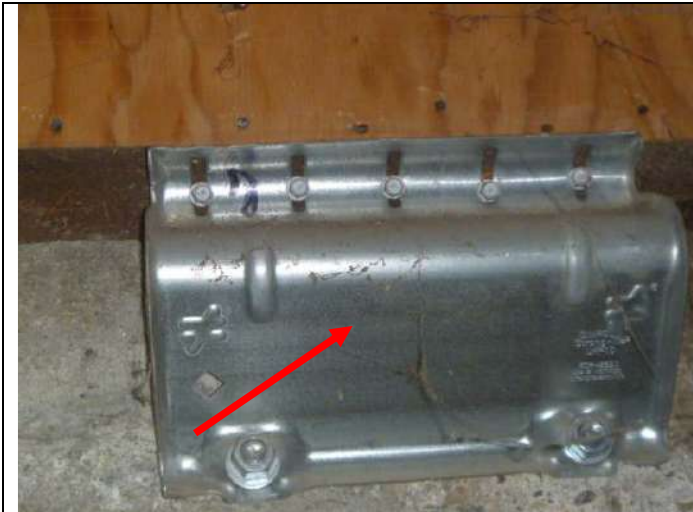
Retrofit foundation anchor plate.
