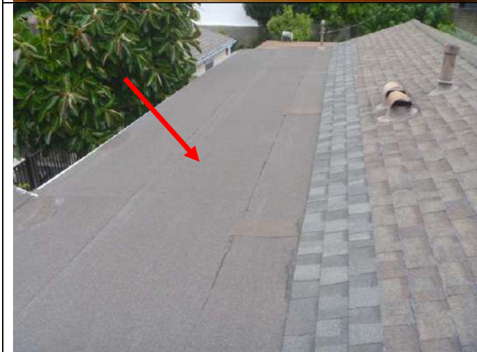
Torch down roofing.
