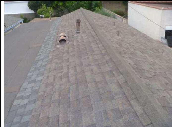
Composition shingle roofing.
