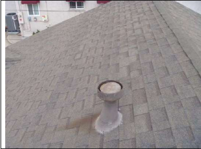
Composition shingle roofing.
