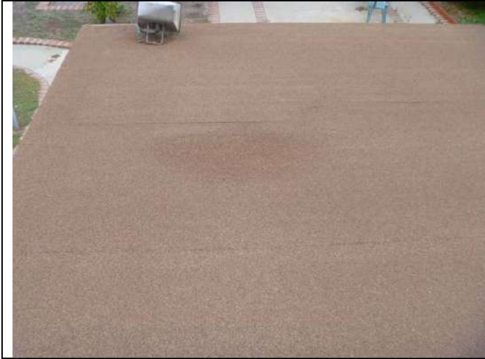
Rear patio covering roof.
