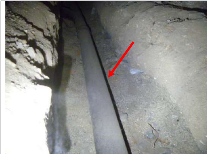
Replacement ABS drain piping.
