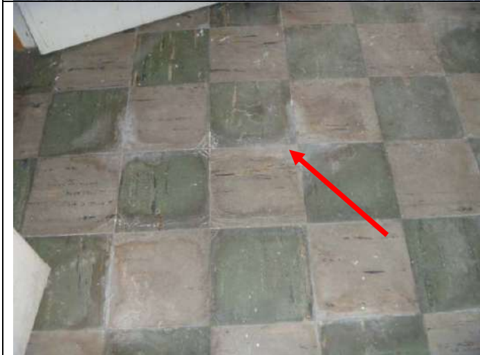
VCT flooring, with possible asbestos content, in the garage side room.
