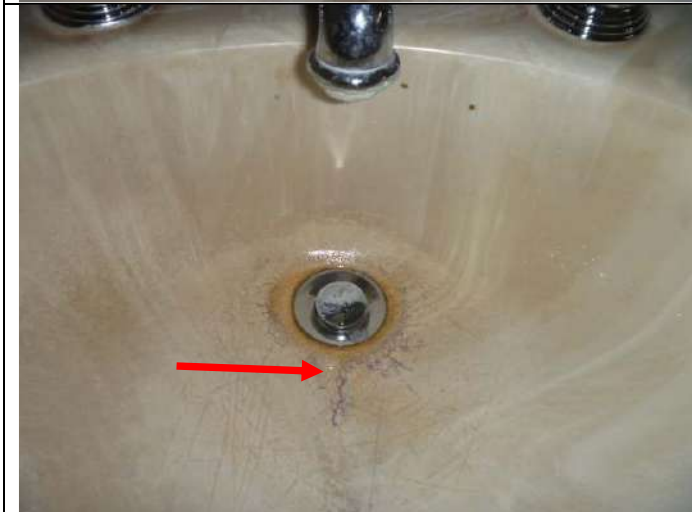
Discoloration in the rear bathroom right sink.
