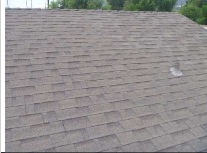
Composition shingle roofing.
