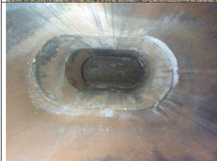
View down the chimney flue.
