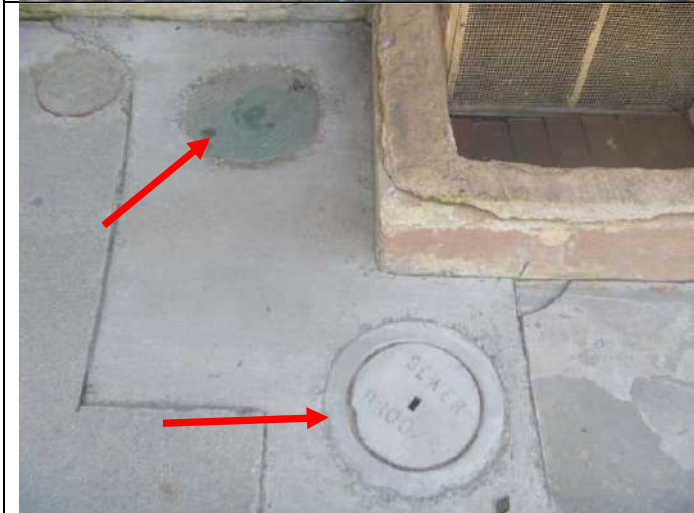
Drain cleanouts at the east side walkway.
