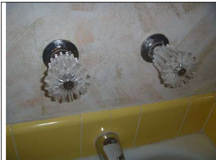
Full bathroom older tub fixtures.
