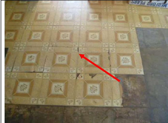
Old vinyl flooring tiles in the garage.
