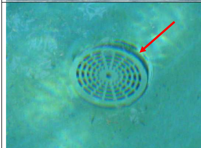
Pool old flat and loose drain cover.
