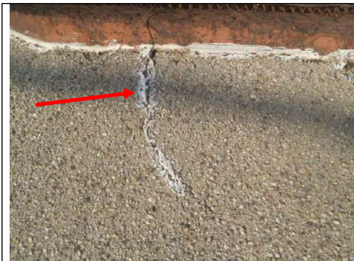
Sealed cracks in the mortar crown.
