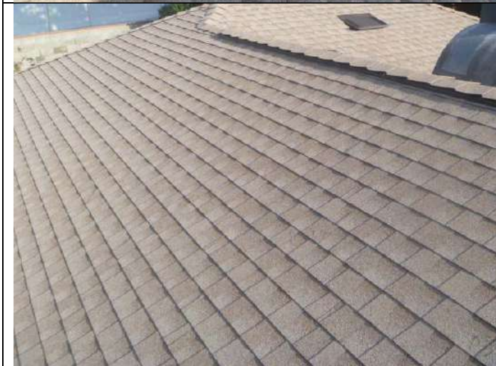
Composition shingle roofing.
