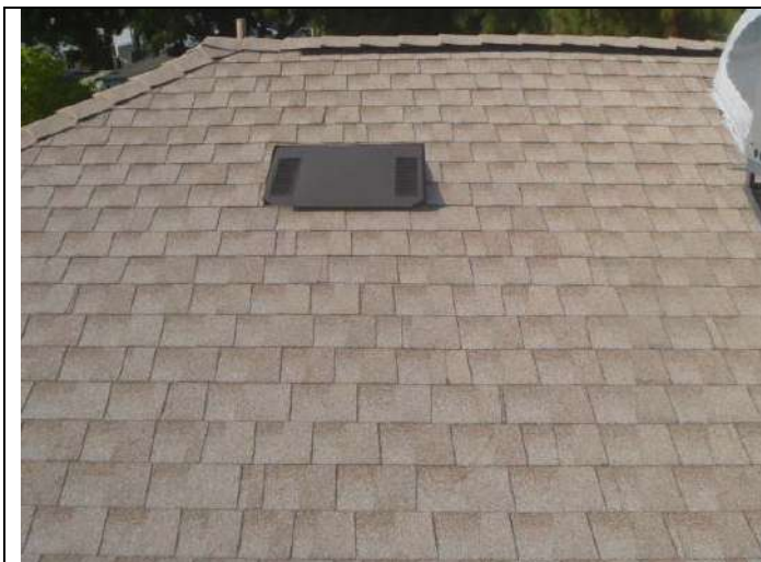
Composition shingle roofing.
