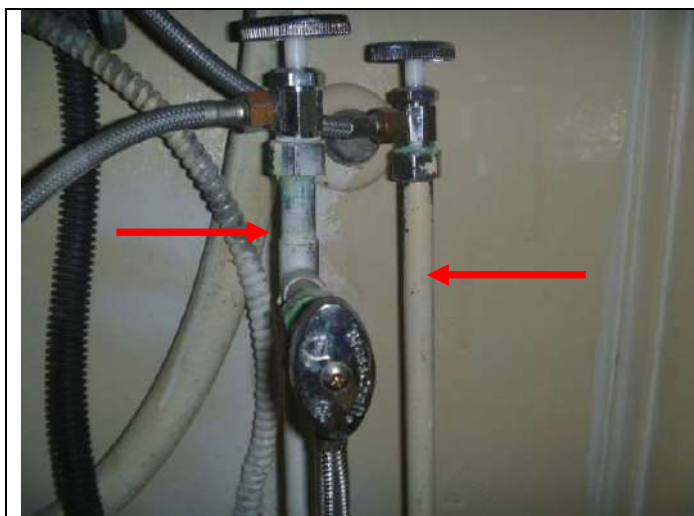
Replacement copper water piping below the kitchen sink.
