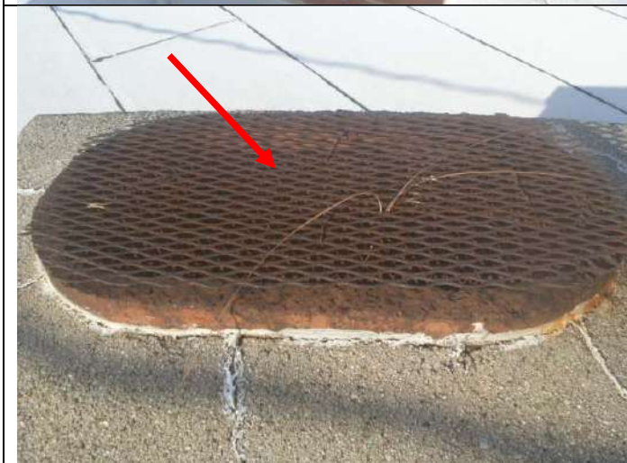
Flat type spark arrestors (vs. a spark arrester/rain cap).
