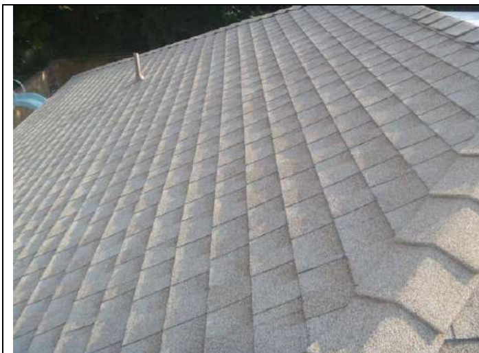
Composition shingle roofing.
