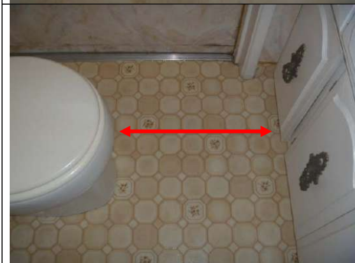
Full bathroom somewhat limited clearance between the toilet and the sink cabinet.
