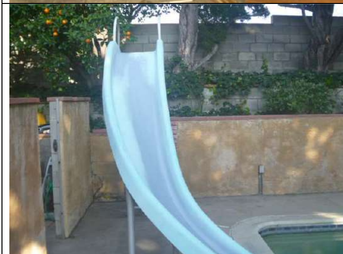
Pool slide (possibly required to be removed).
