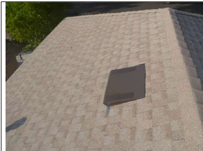
Composition shingle roofing.
