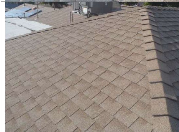
Composition shingle roofing.
