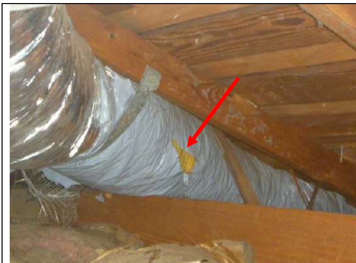
Old heating/air conditioning duct leading to the family room register.
