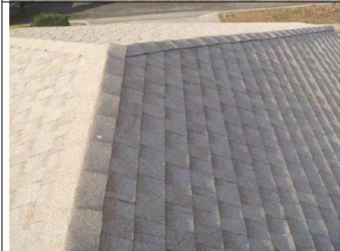
Composition shingle roofing.
