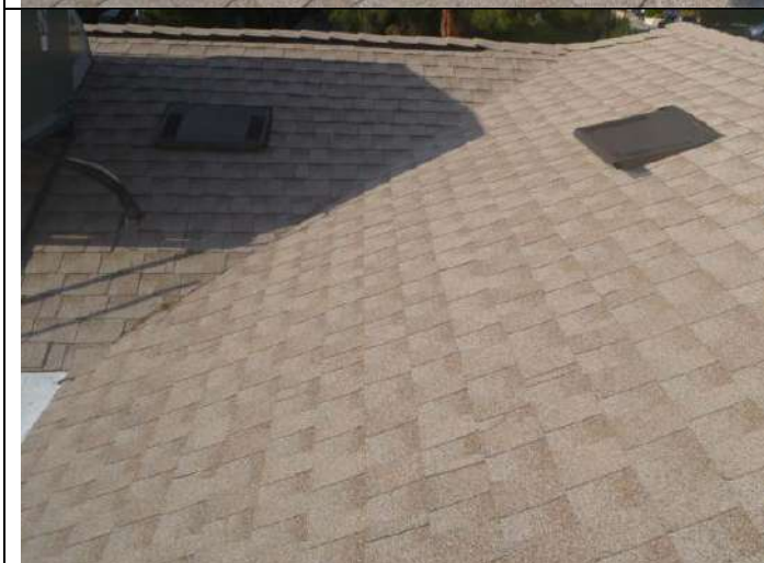
Composition shingle roofing.
