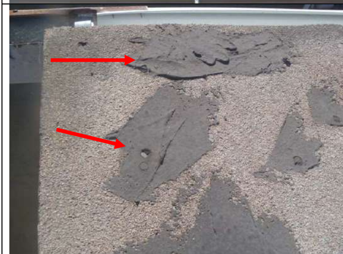
Irregular sealant on the storage structure roof.
