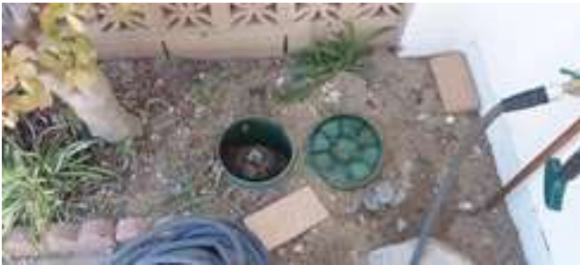
Cleanout used for today's inspection.
