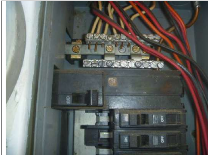
A closer view of the main breaker.
