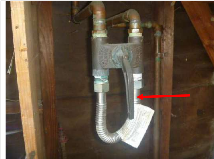
Hookups for a water softener at the left front interior of the garage.
