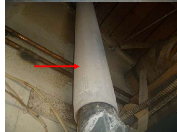
Heater transite vent pipe.
