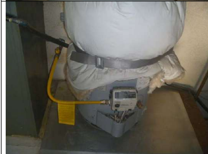
Water heater lower section. Note: There is no catch pan.
