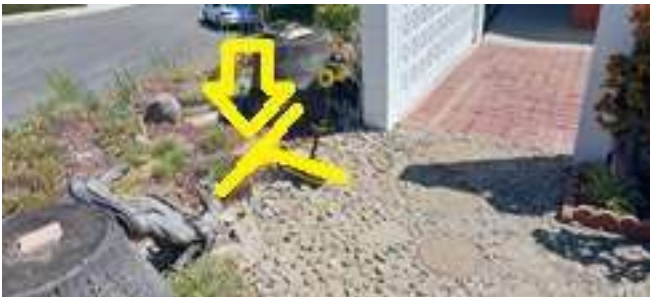
Install new cleanout here. Depth about 3 ½'. Install bull horns style so that you can look back toward the main house as well.
