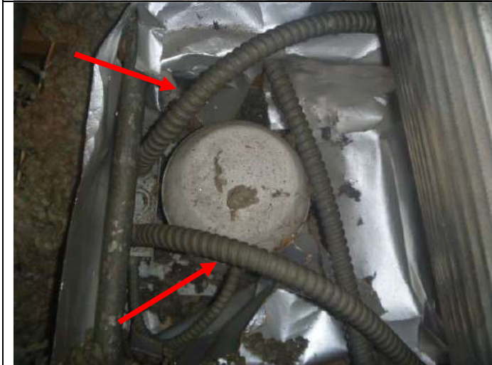
Flexible conduit wiring. Note: The majority of the wiring is this type.
