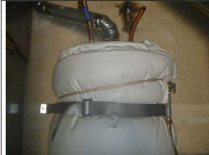
Water heater upper section. Note: The seismic bracing is installed (vs. under) in the insulation blanket.
