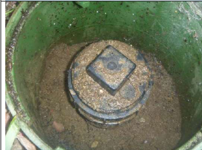
Main drain cleanout at the southeast exterior of the garage.
