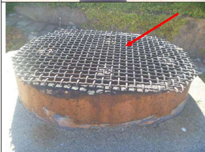
Flat type spark arrestor (vs. a spark arrestor/rain cap).
