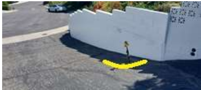
Path of main line. Depth about 4'.
