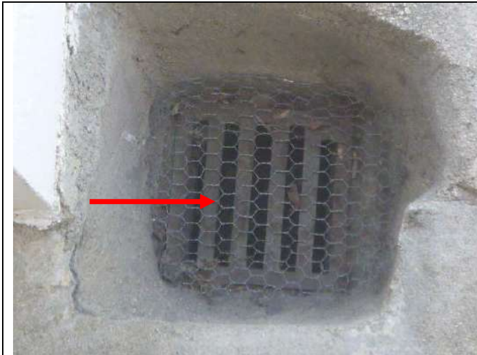
An exterior surface drain (at the center front).
