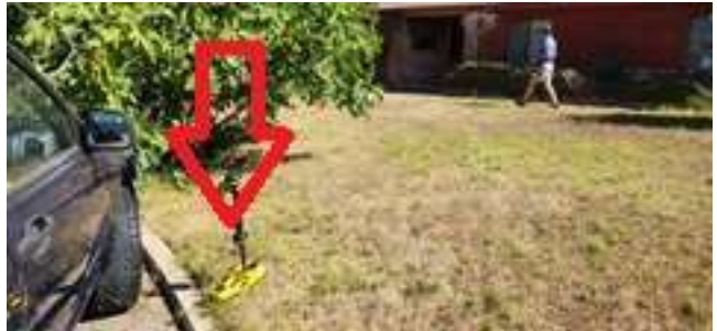
Sewer line exits property about 7 feet deep
