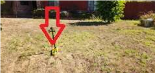
Line drops deeper and turns toward street
