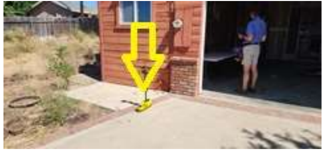
Furthest point reached from ADU roof vent. Good spot for cleanout installation. About 4 feet deep
