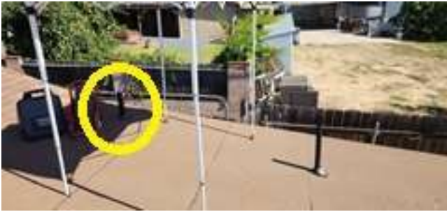
2 inch roof vent used for inspection from ADU
