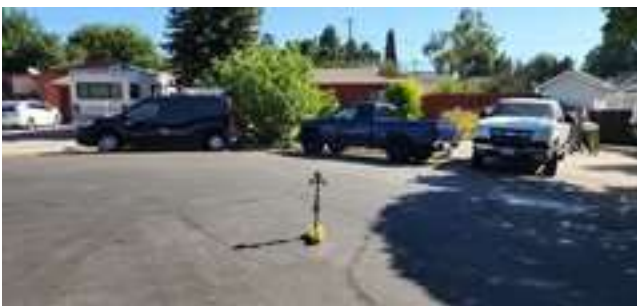
Connection to city sewer line about 10 feet deep
