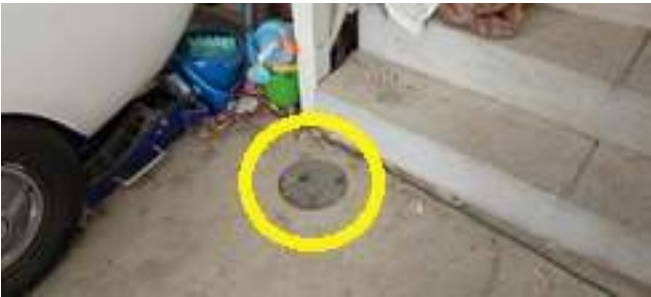
Main sewer cleanout used for today’s inspection.
