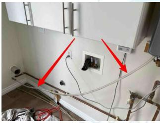
There does not appear to be the required bonding connection between the water pipes and the gas pipe.
