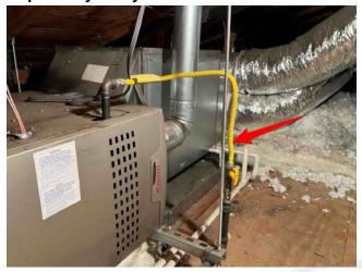
There are areas with hard piped, gas lines, and no flexible sections of gas piping. Flexible sections of piping are recommended to allow for movement in the case of an earthquake at the water heater.
