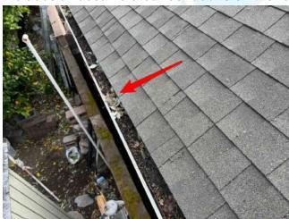
All of the house and portions of the garage building have no guttering system to take the roof water properly off the structure.
