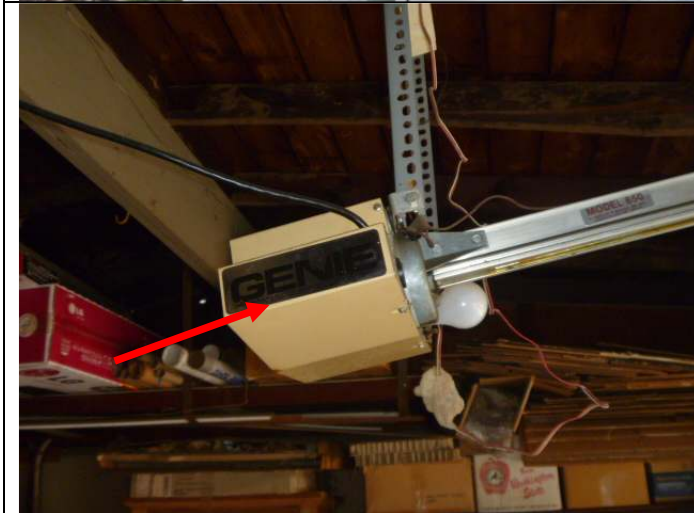
Old garage door opener.
