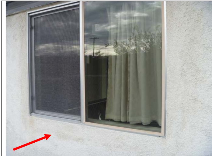
Stucco repair at the kitchen rear window.
