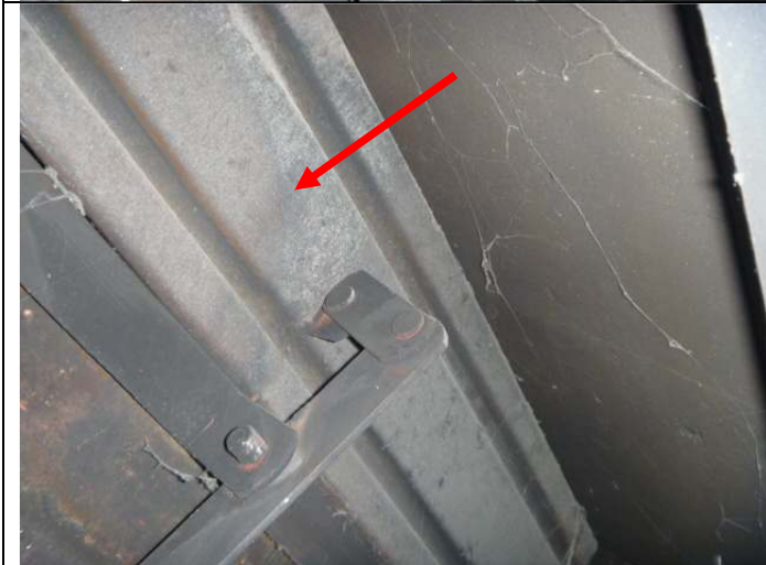
Fireplace damper in the closed position.
