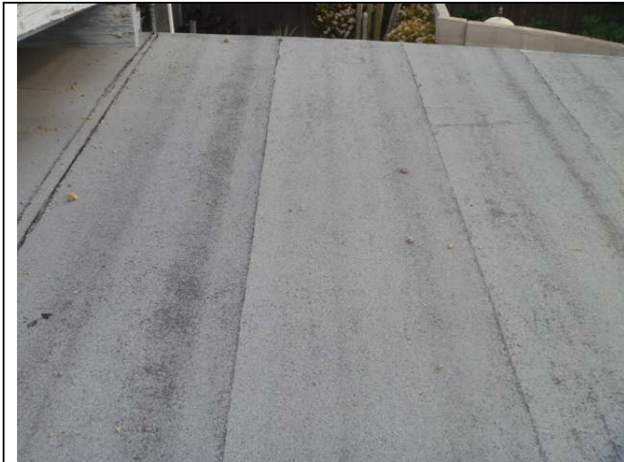
Patio room roof.
