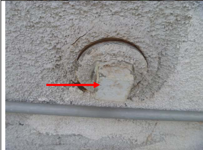
Drain cleanout at the lower north exterior wall.
