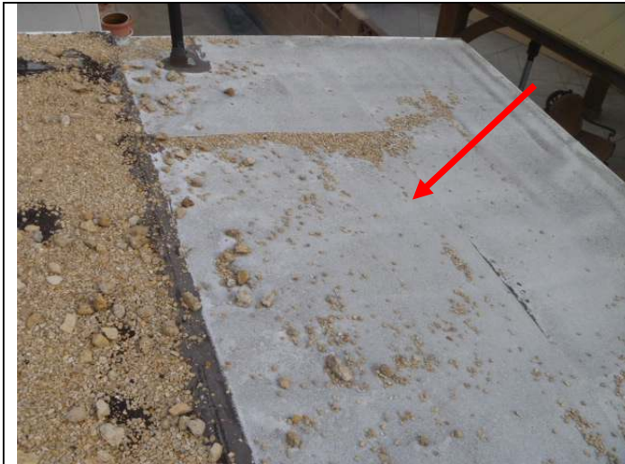
Rolled composition or similar roofing over the full bathroom.
