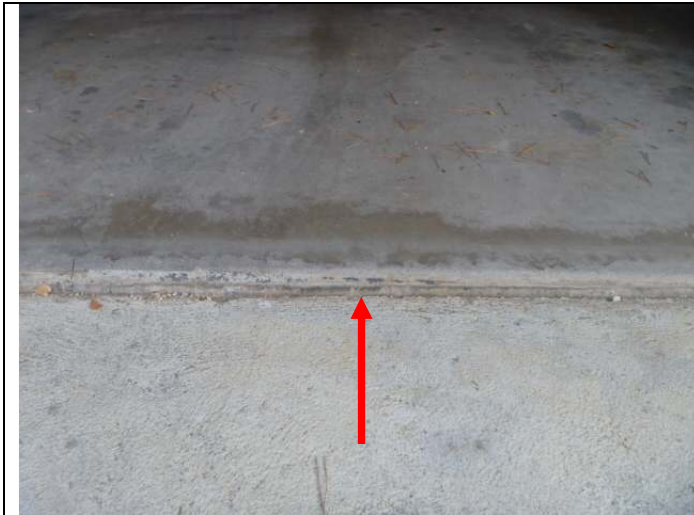
Step along the front of the garage slab floor.
